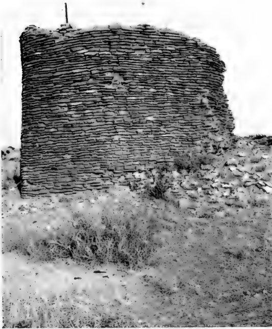
Remains of Spanish mission church at Pueblo San Cristóbal. Built probably during the first half of the seventeenth century and abandoned in 1680
